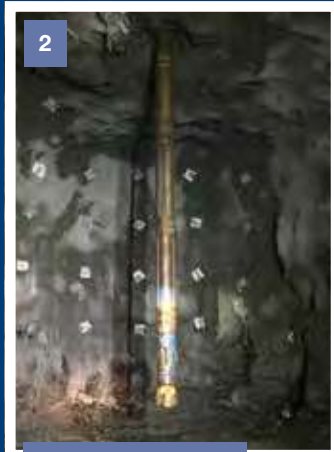
Pilot hole breakthrough.
